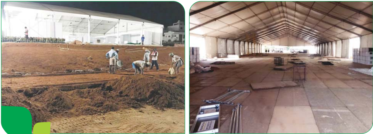
Figure 3: During: The venue in the works
